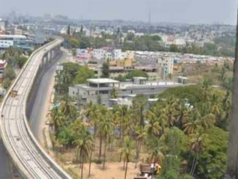
Empty Bangalore Mysore Road and Metro track in Bangalore
