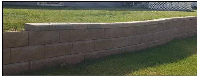
Photo 4.7.4.1-1 Stacked stone retaining wall
