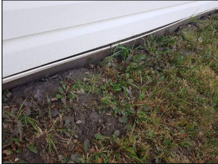
Photo 4.1.1.1-4 Typical level of grade to foundation wall
