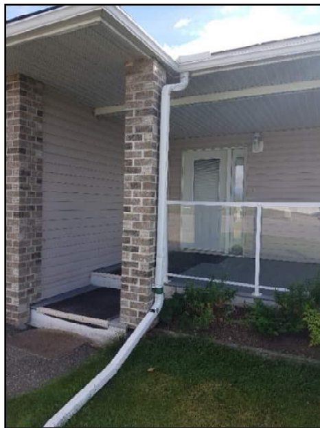
Photo 4.2.1.2-1 Typical stone column
