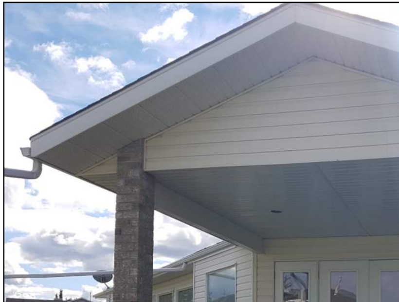
Photo 4.2.3.3-1 Typical fascia cladding
