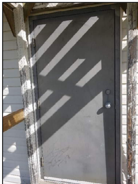
Photo 4.2.2.2-3 Metal exit door
