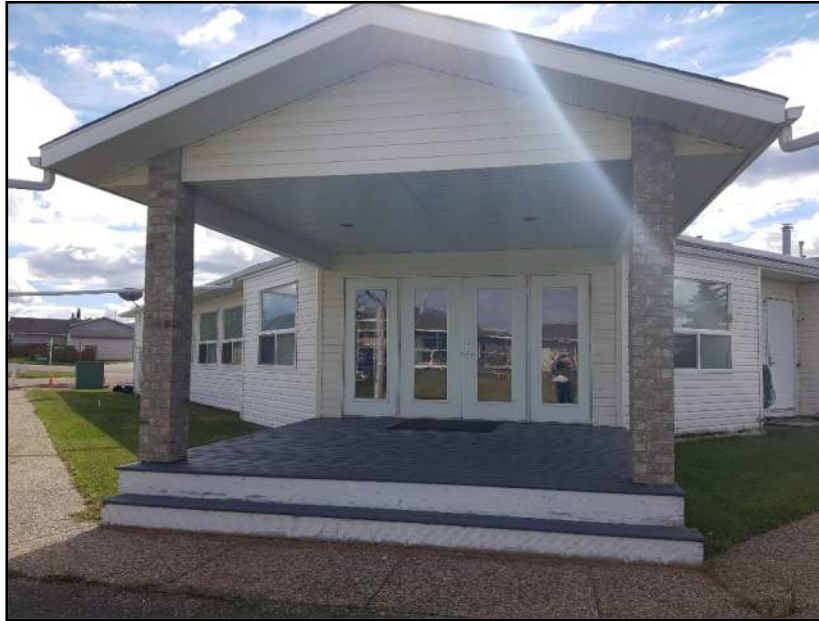
Photo 4.7.2.1-2 Wood deck at sunroom
