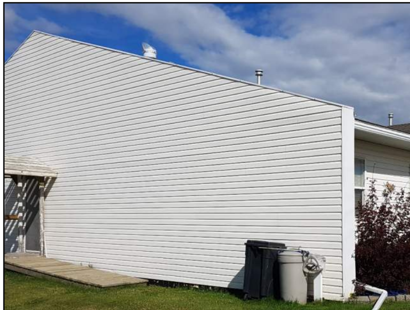
Photo 4.2.1.1-1 Typical vinyl siding
