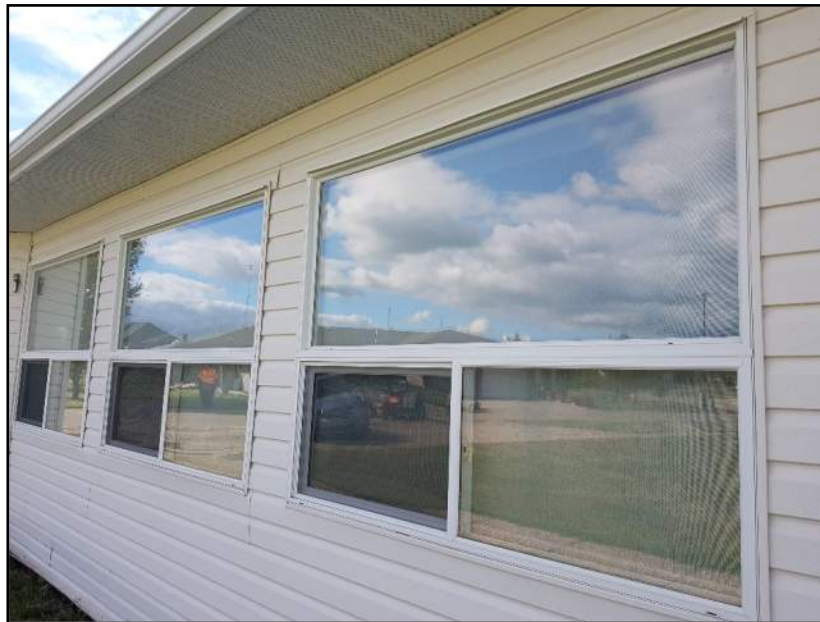
Photo 4.2.2.1-1 Typical vinyl windows at the octuplex common areas
