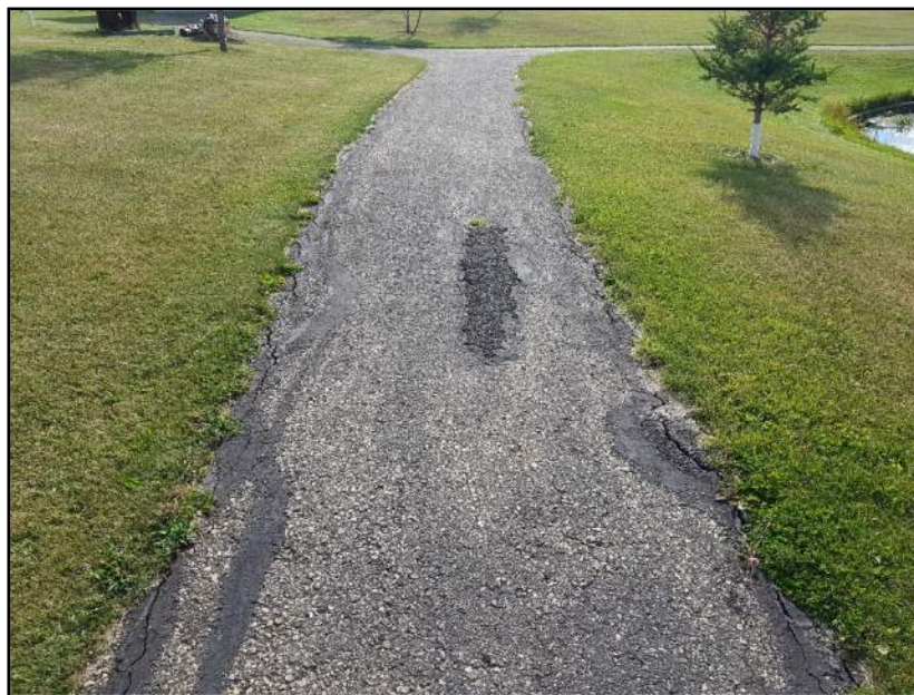
Photo 4.7.1.3-1 Typical asphalt walkway
