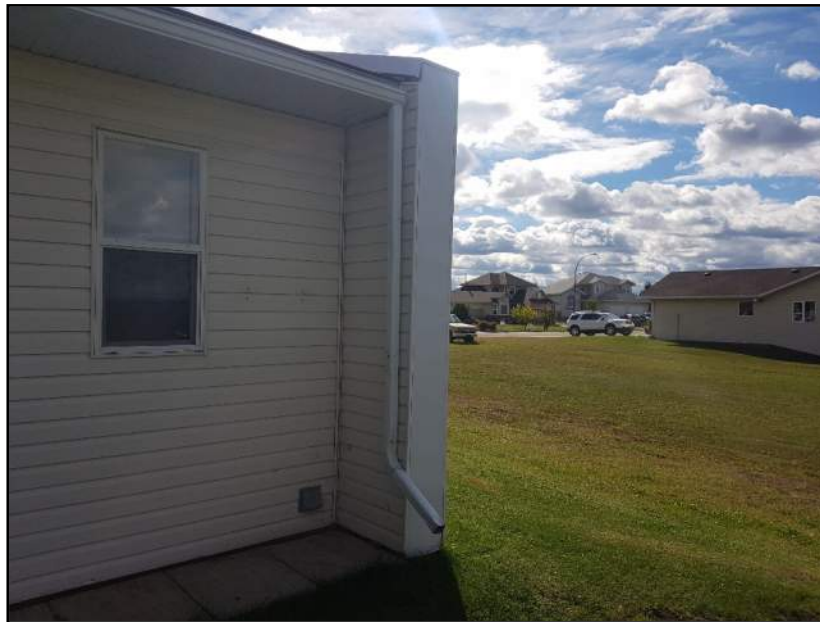
Photo 4.2.3.2-1 Typical eavestroughs and downspout
