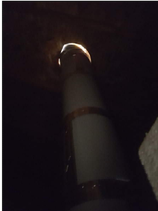
Photo 4.2.3.1-3 Unsealed vent stack
