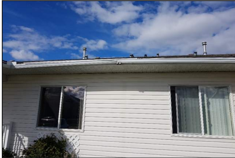
Photo 4.1.2.1-2 Shifted soffit
