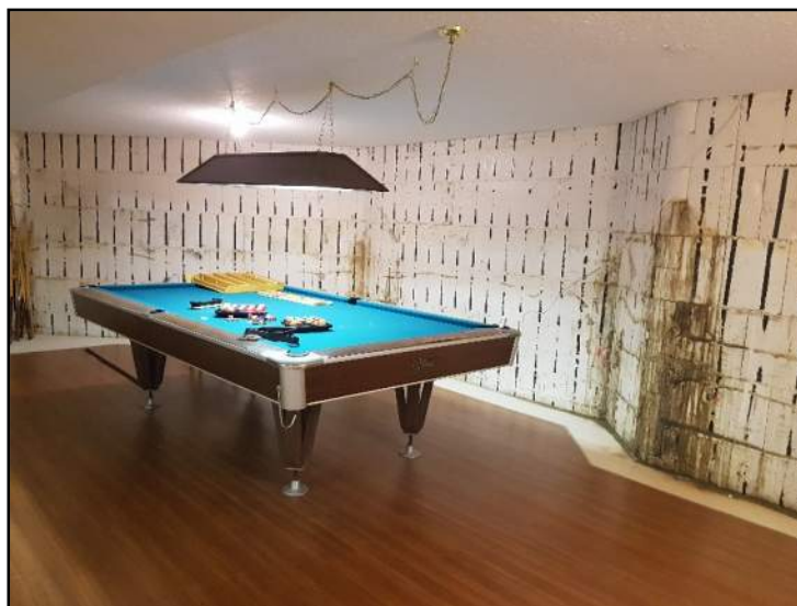
Photo 4.3.1.1-4 Basement amenity space
