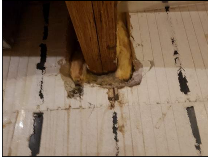
Photo 4.1.1.1-2 Typical beam pocket condition
