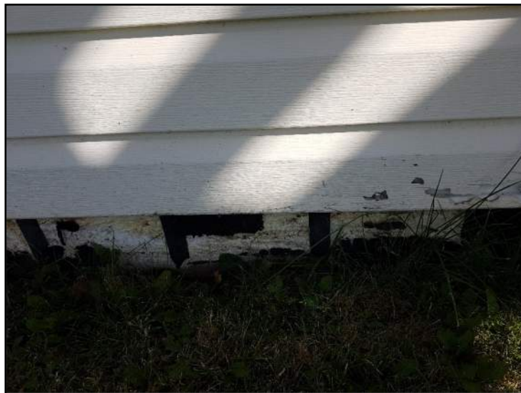
Photo 4.1.1.1-3 Typical exposed waterproofing on IFC foundation
