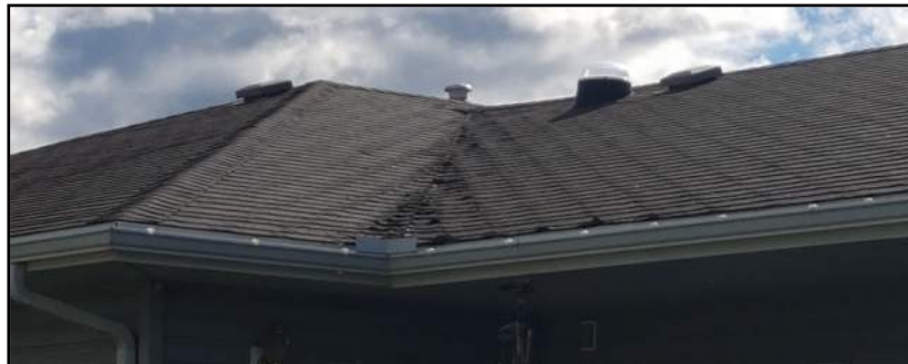
Photo 4.2.3.1-1 Typical 2000 / 2004 roof valleys
