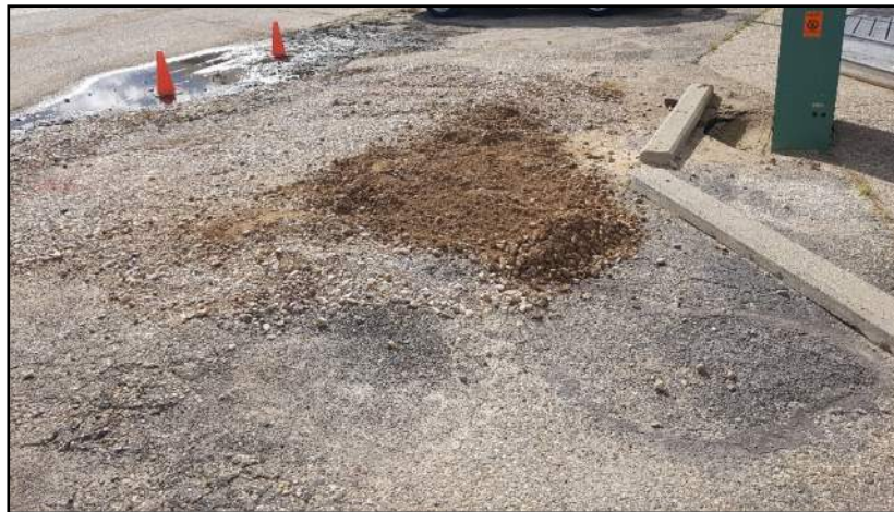
Photo 4.7.1.1-1 Typical paving condition
