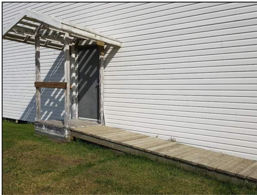
Photo 4.7.2.1-1 Wood deck at corridor entrance
