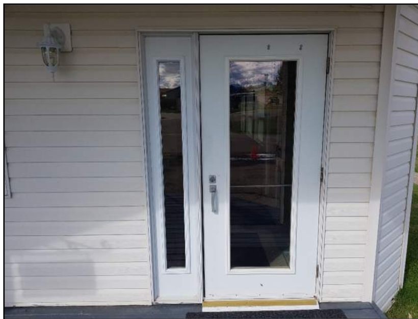
Photo 4.2.2.2-1 Main entrance door
