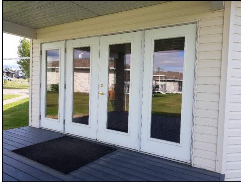
Photo 4.2.2.2-2 Rear deck sunroom doors
